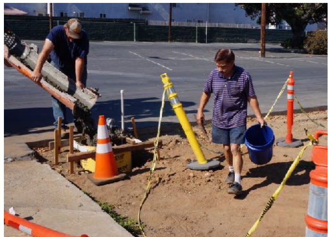
Setting concrete bases for new light poles & shade cloth anchors!
